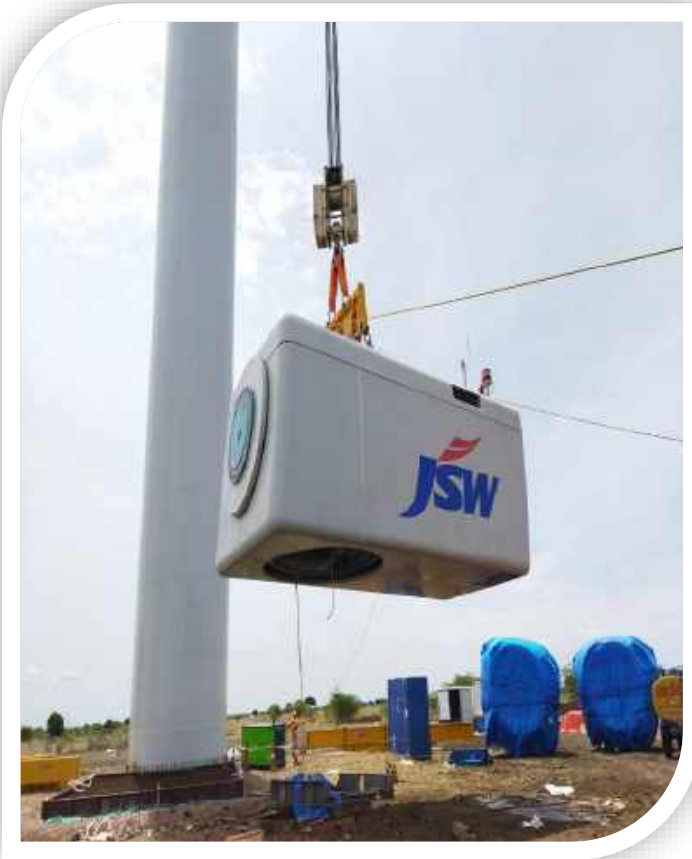
Blades and WTG erection followed by progressive commissioning (27MW commissioned)
