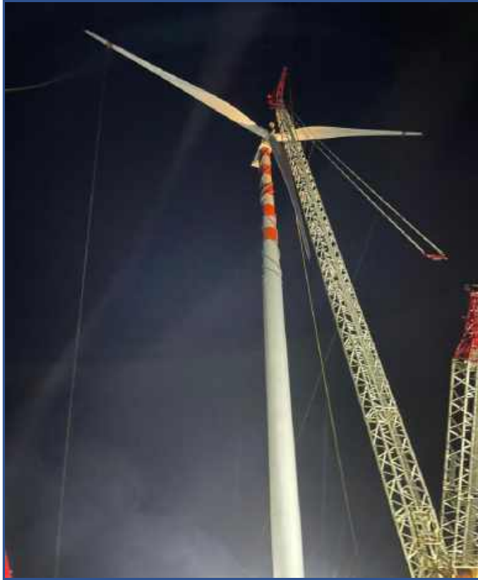
WTG Erection work in progress
