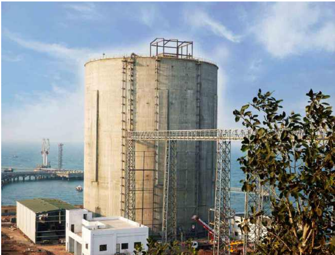
Completed the construction of 45,000 MT Ash Silo of JSW Energy at Ratnagiri JSW Port
