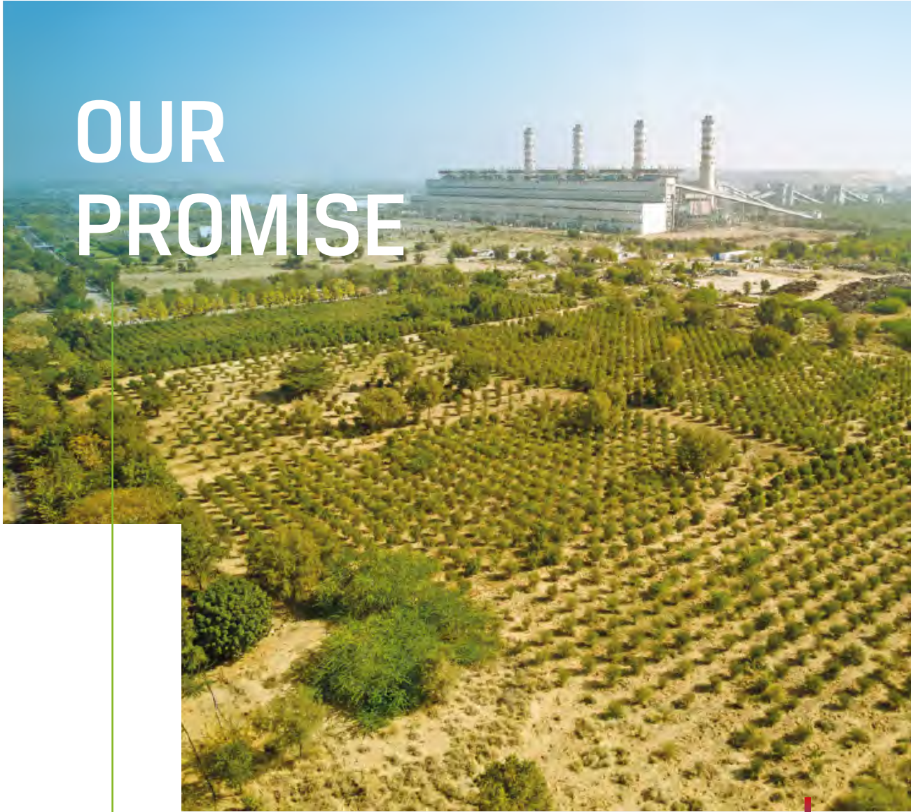
Barmer Thermal Plant
