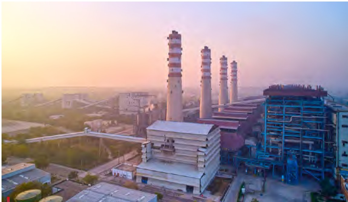
Thermal Power Plant, Barmer
