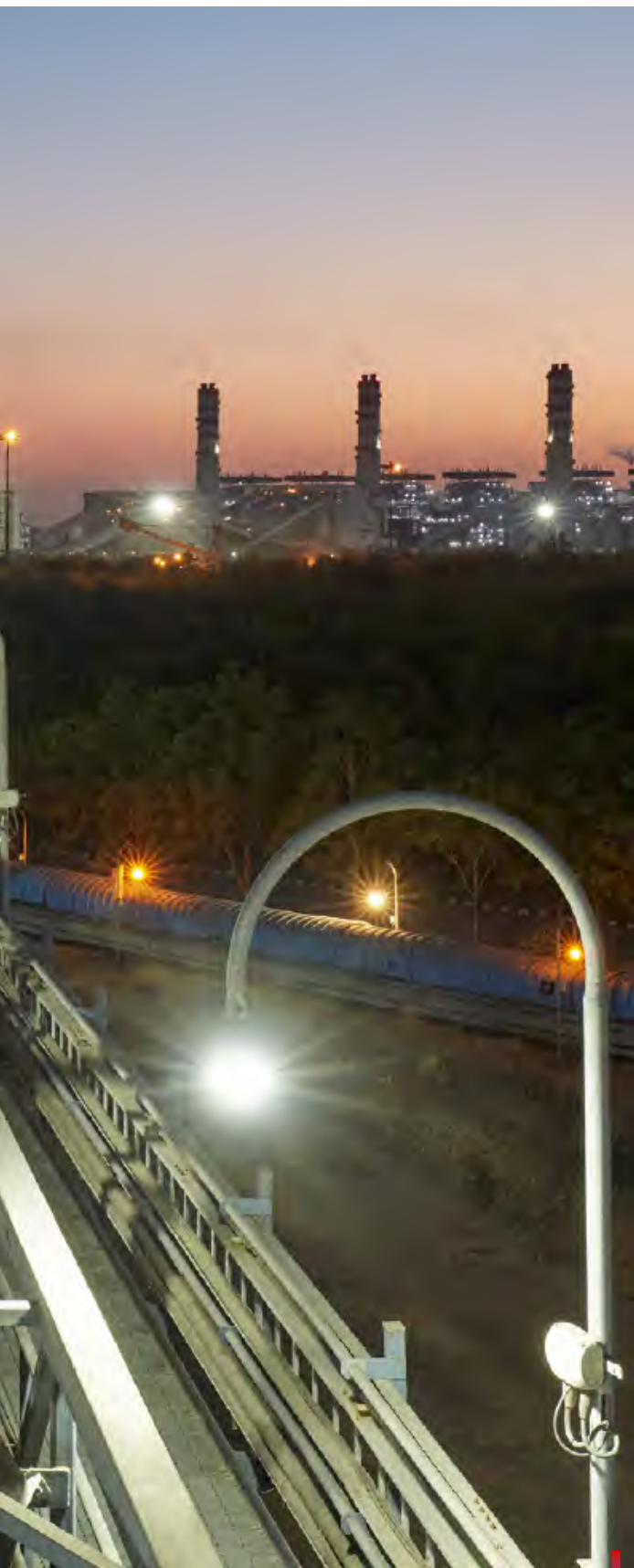
Barmer Power Plant
