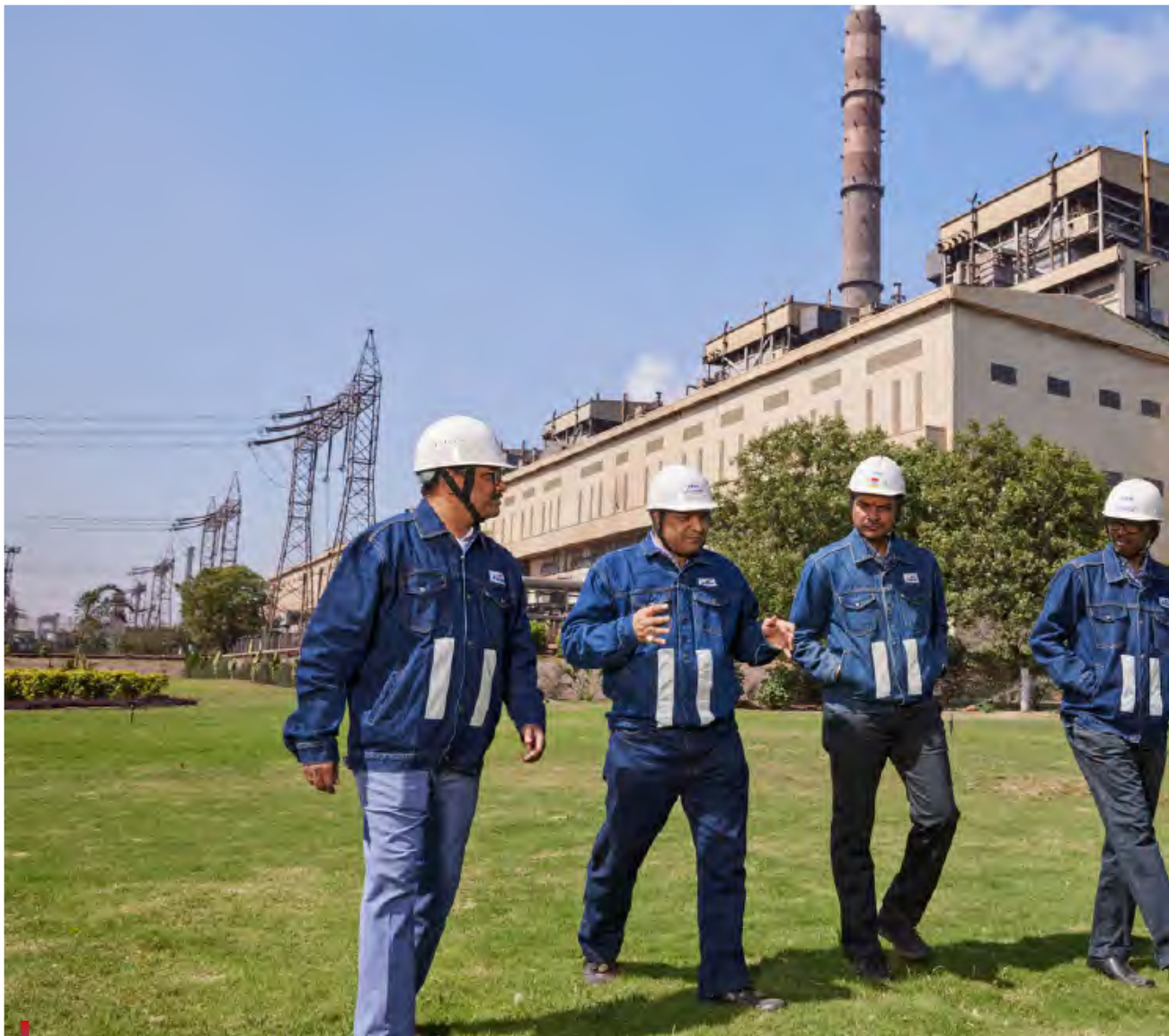
JSW Energy, Vijayanagar
