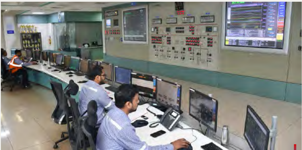
Thermal Power Plant, Ratnagiri
