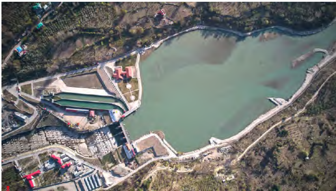
Hydro Power Plant, Sholtu
