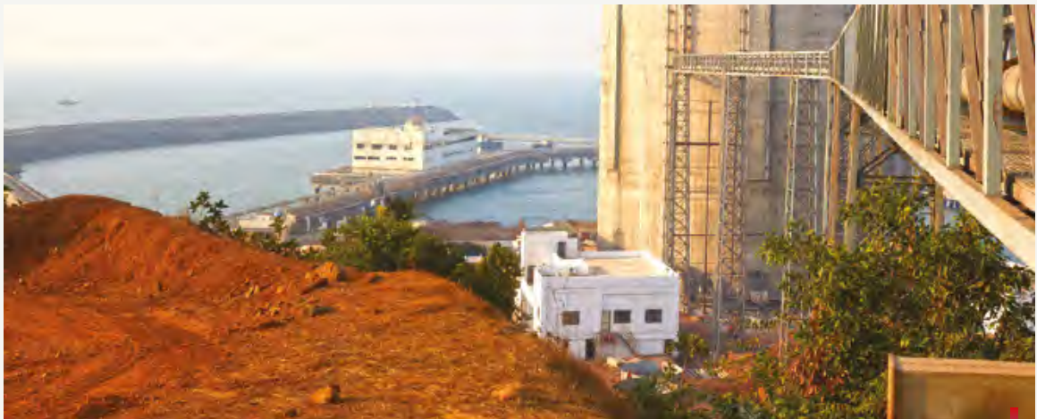
Fly Ash Silo at Ratnagiri Plant
