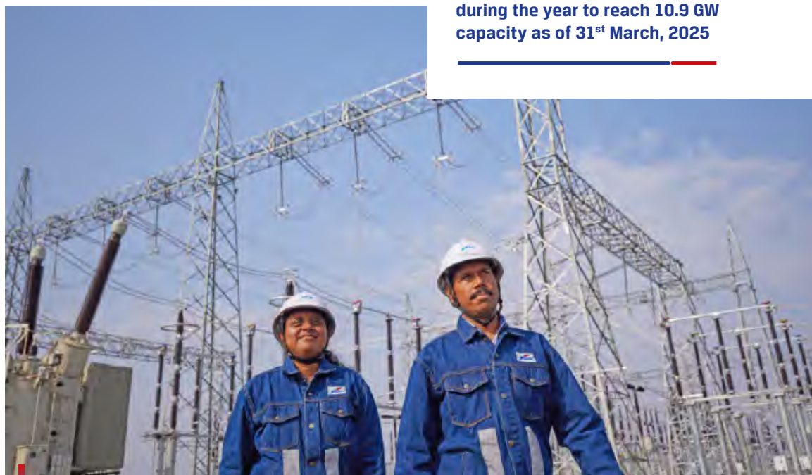
Solar Power Plant, Vijayanagar
