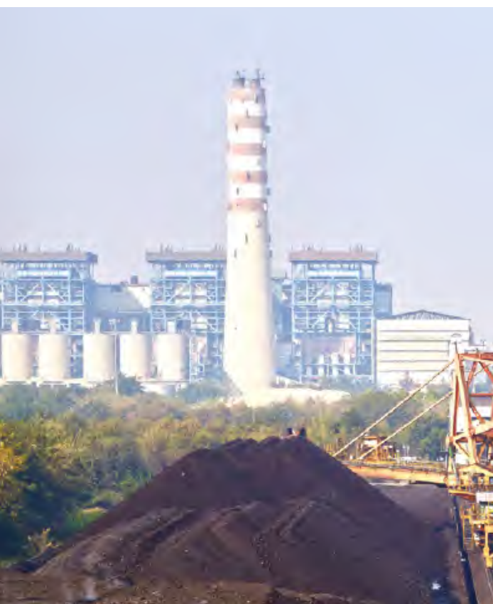
Power Plant, Utkal
