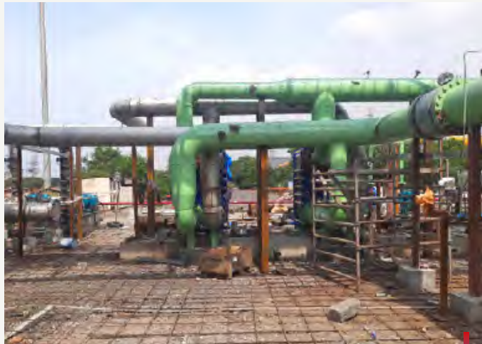
Green Hydrogen Plant, Underconstruction at Vijayanagar
