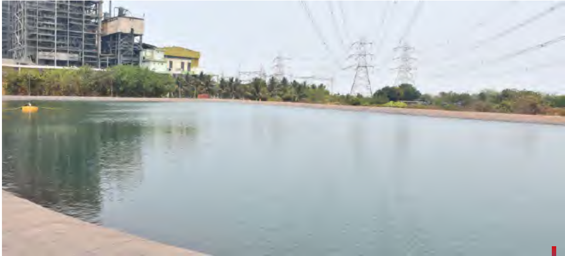
New Water Reservoir at Ratnagiri Plant
