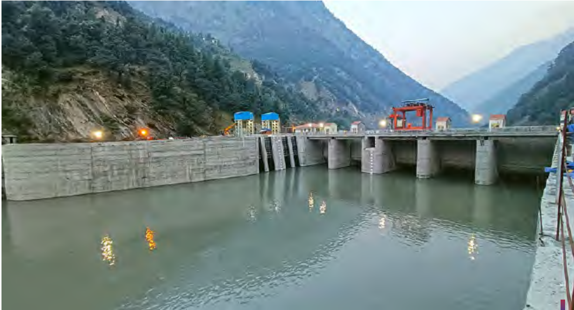
Barrage, Kutehr Hydro Project
