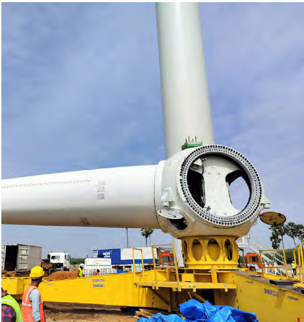
Wind Turbine Construction at Tuticorin Project
