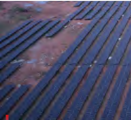
Solar Plant, Vijayanagar
