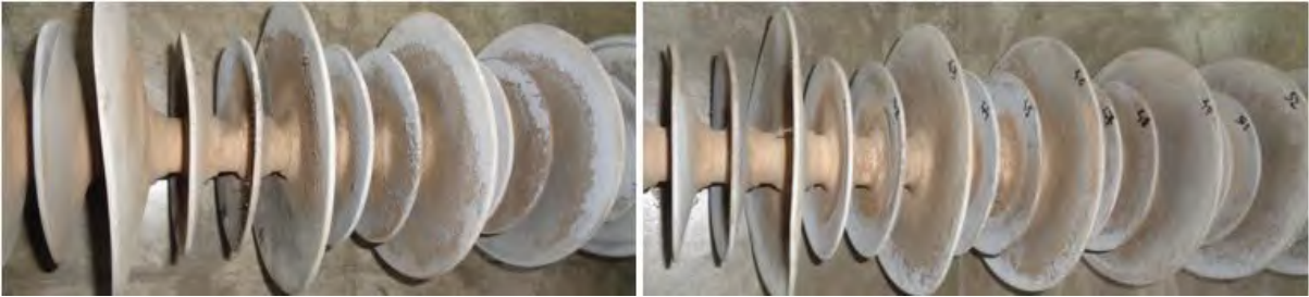
Figure 2.39: As received working insulator (SRI-5) received for analysis
