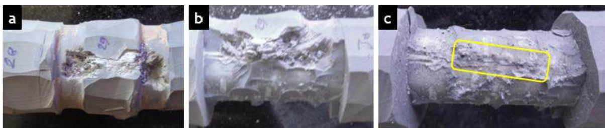
Figure 2.44: a) Punctured sheath, b) degraded silicone rubber and c) composite rod degradation found localised (highlighted in yellow border)
