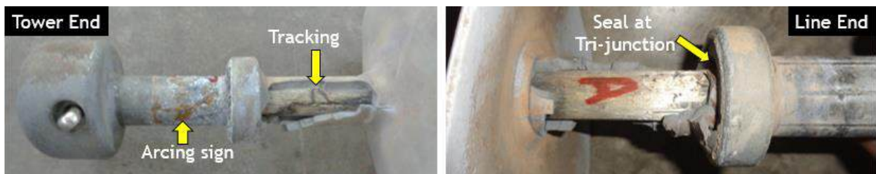
Figure 2.3: As received failed insulator (SRI-1) at the line end and tower end. Yellow arrow indicate arcing damage to the tower end metallic end fitting
