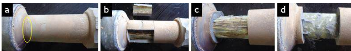
Figure 2.27: a) Crack near the tri-junction, b) cut in silicone rubber, c) degraded composite rod visible and d) back side of same section the composite rod was intact
