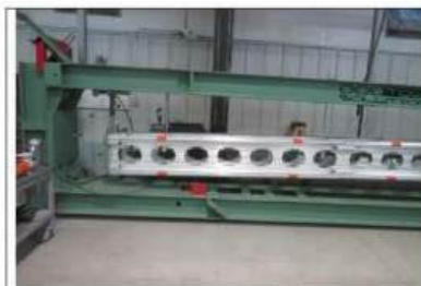
The column has bended
