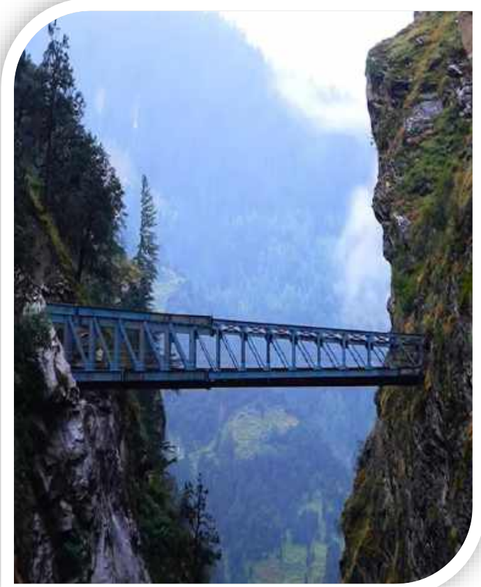
Steel Cantilever Bridge
