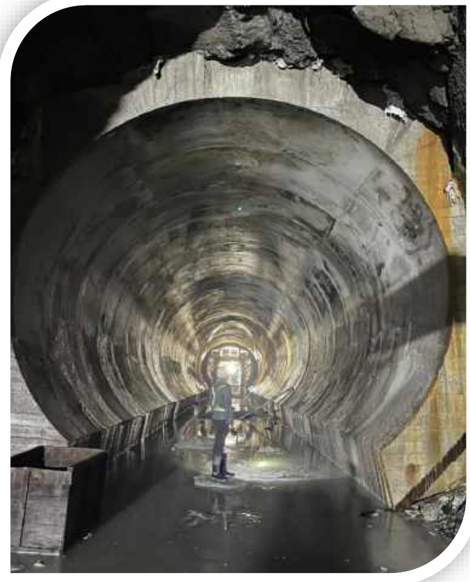
HRT Gantry Concrete Lining
