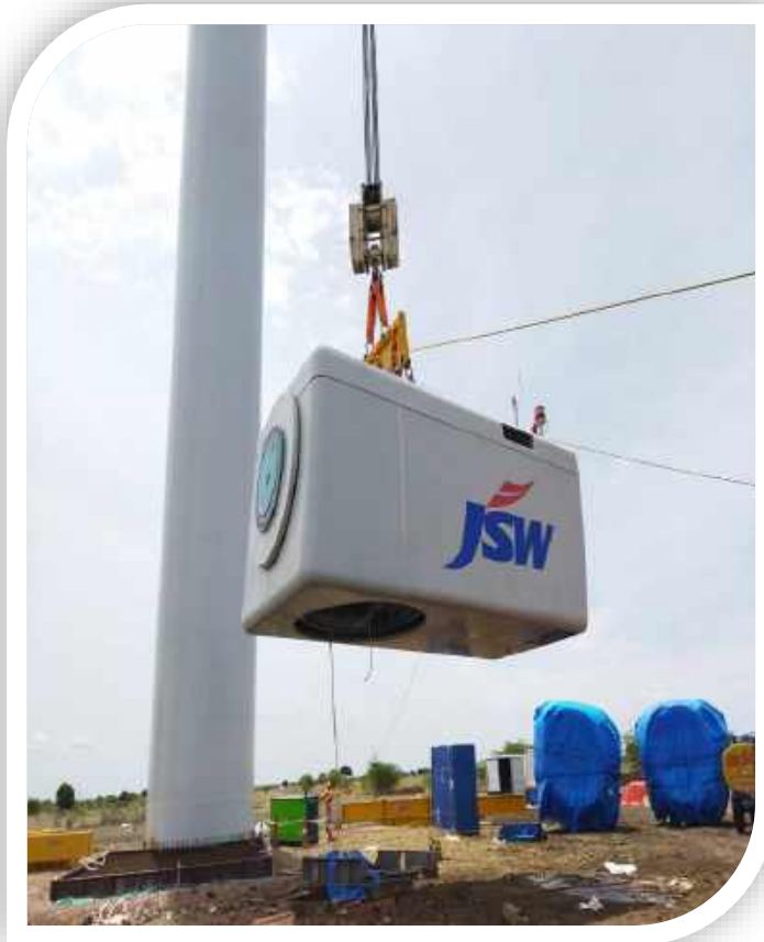
Nacelle and WTG erection
