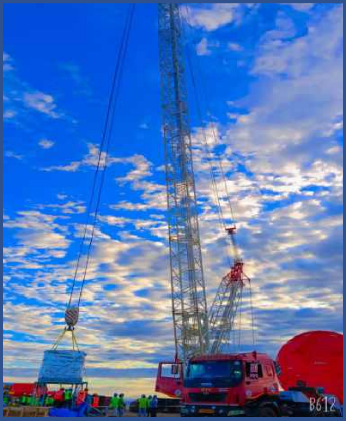
WTG Erection work in progress
