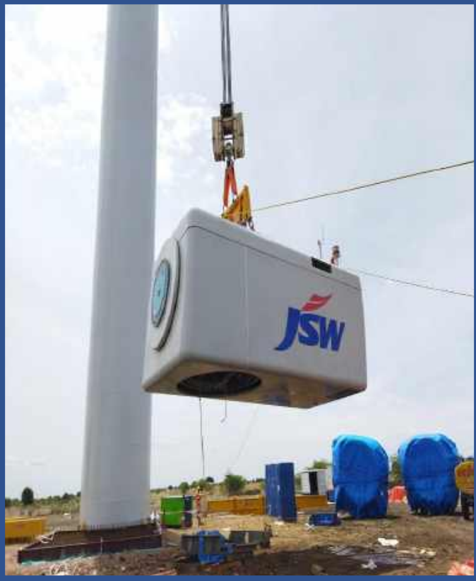
Nacelle Erection work in progress
