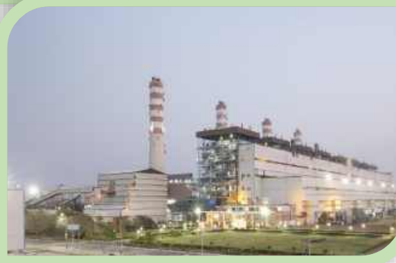
Green Belt & Plantation near Barmer Power Plant
