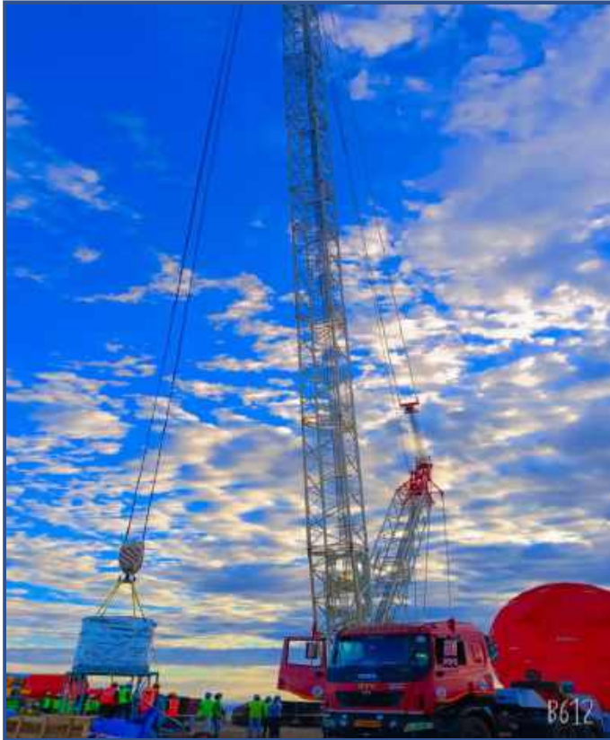
WTG Erection work in progress
