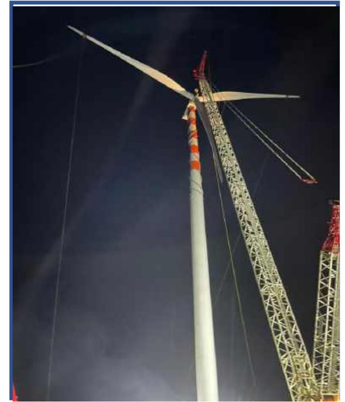
WTG Erection work in progress
