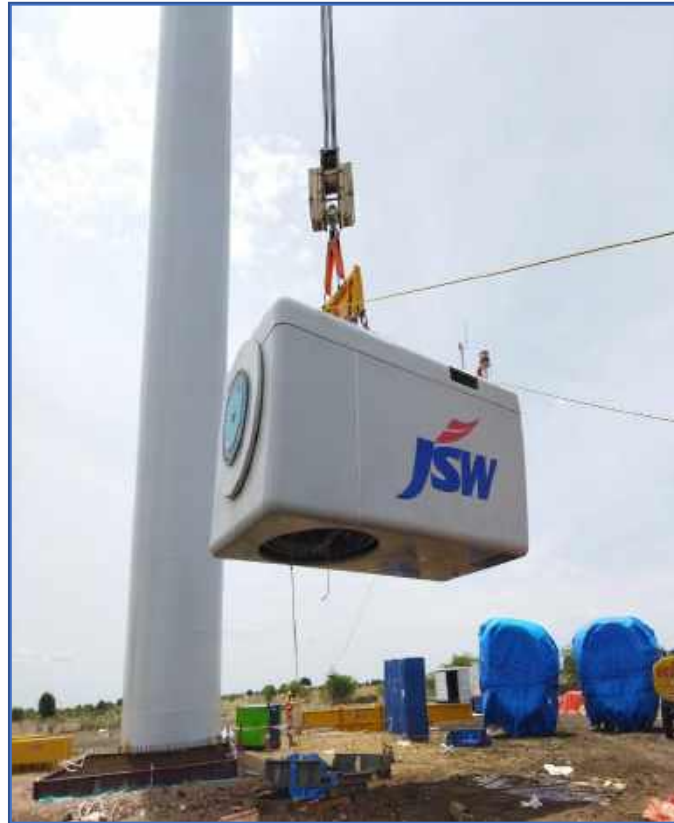
Nacelle Erection work in progress
