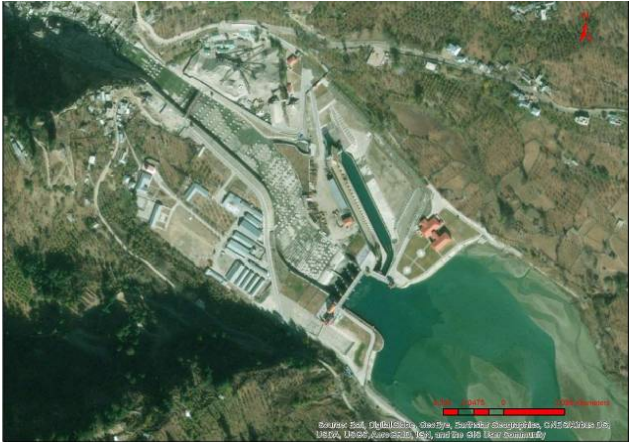
Figure 4.5: Top view of Kuppa Barrage
