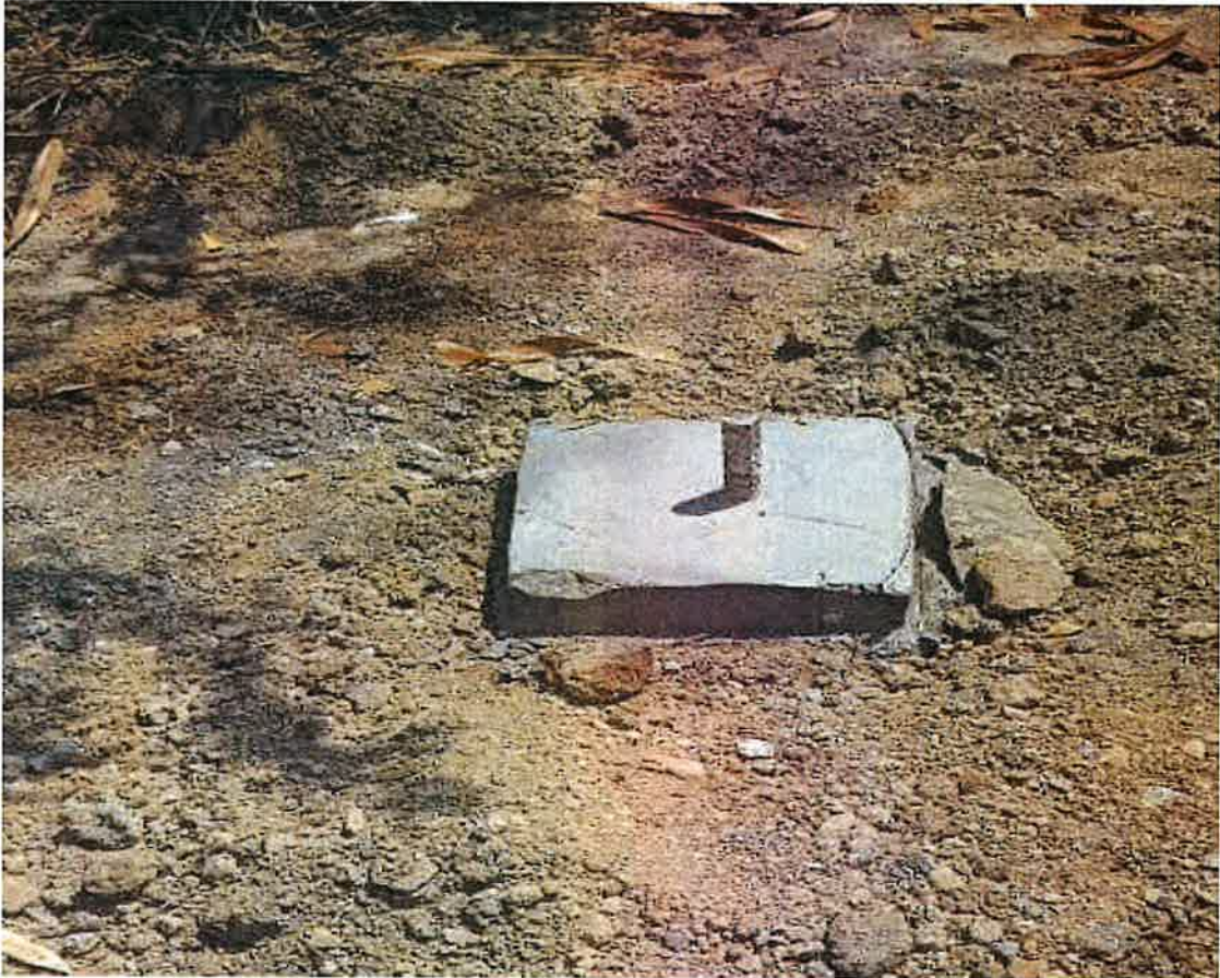
Figure 8. Settlement monitoring point
