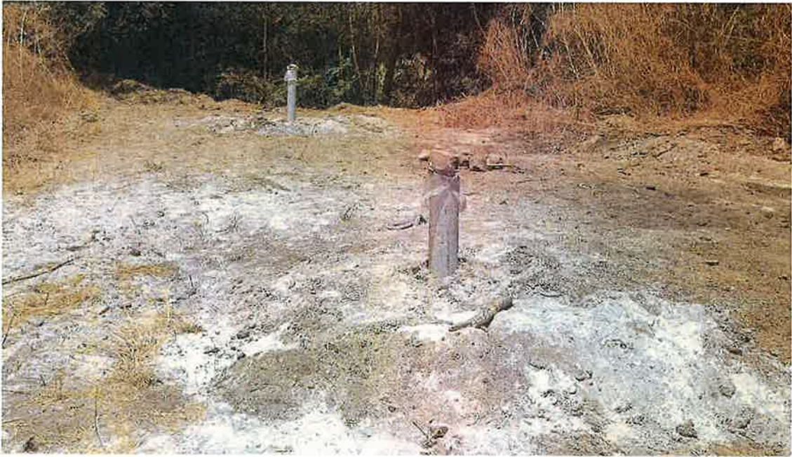
Figure 7. Two seepage monitoring well
