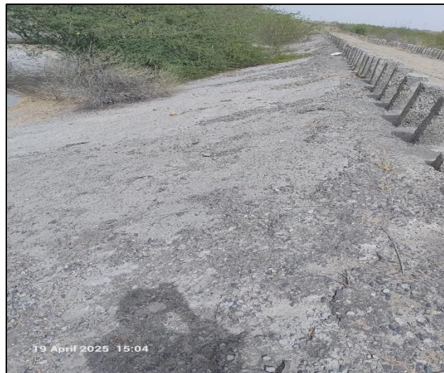
FIG.10: ASH DYKE SLOPE
