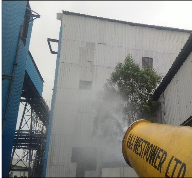
FIGURE 6: SPRINKLER IN ASH DYKE AREA
