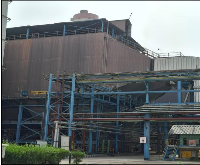
FIGURE 8: ASH COLLECTION- ESP & HOPPER
