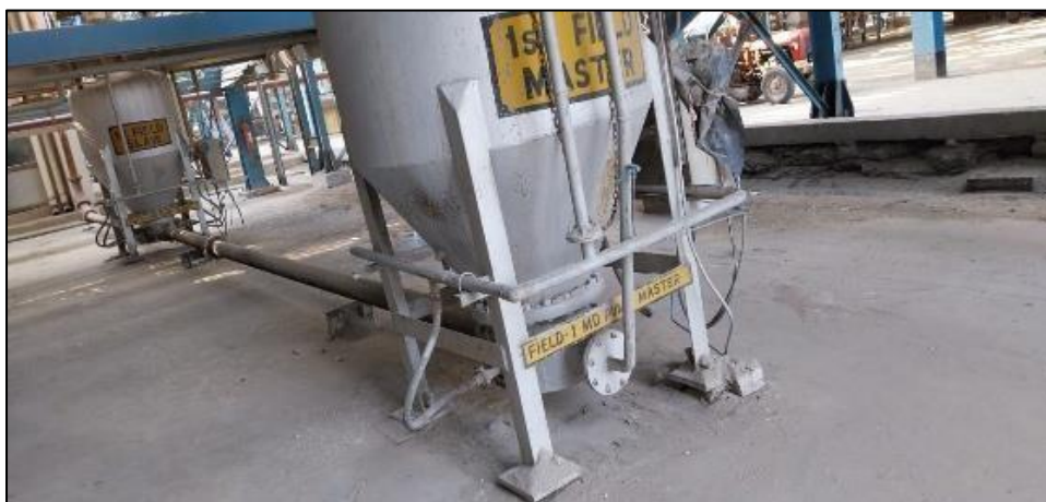
FIGURE 12: ASH TRANSPORT SYSTEM
