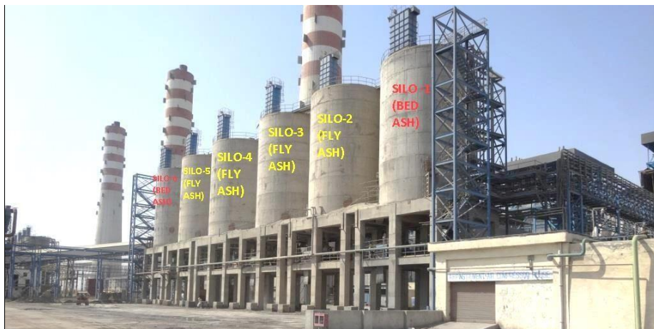
FIGURE 11: ASH STORAGE ONSITE SILOS- FLY ASH AND BOTTOM
