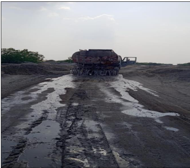
FIGURE 7: WATER SPRAY THROUGH TANKER IN ASH DYKE AREA
