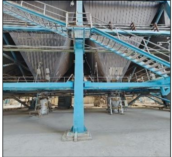
FIGURE 8: ASH COLLECTION- ESP & HOPPER
