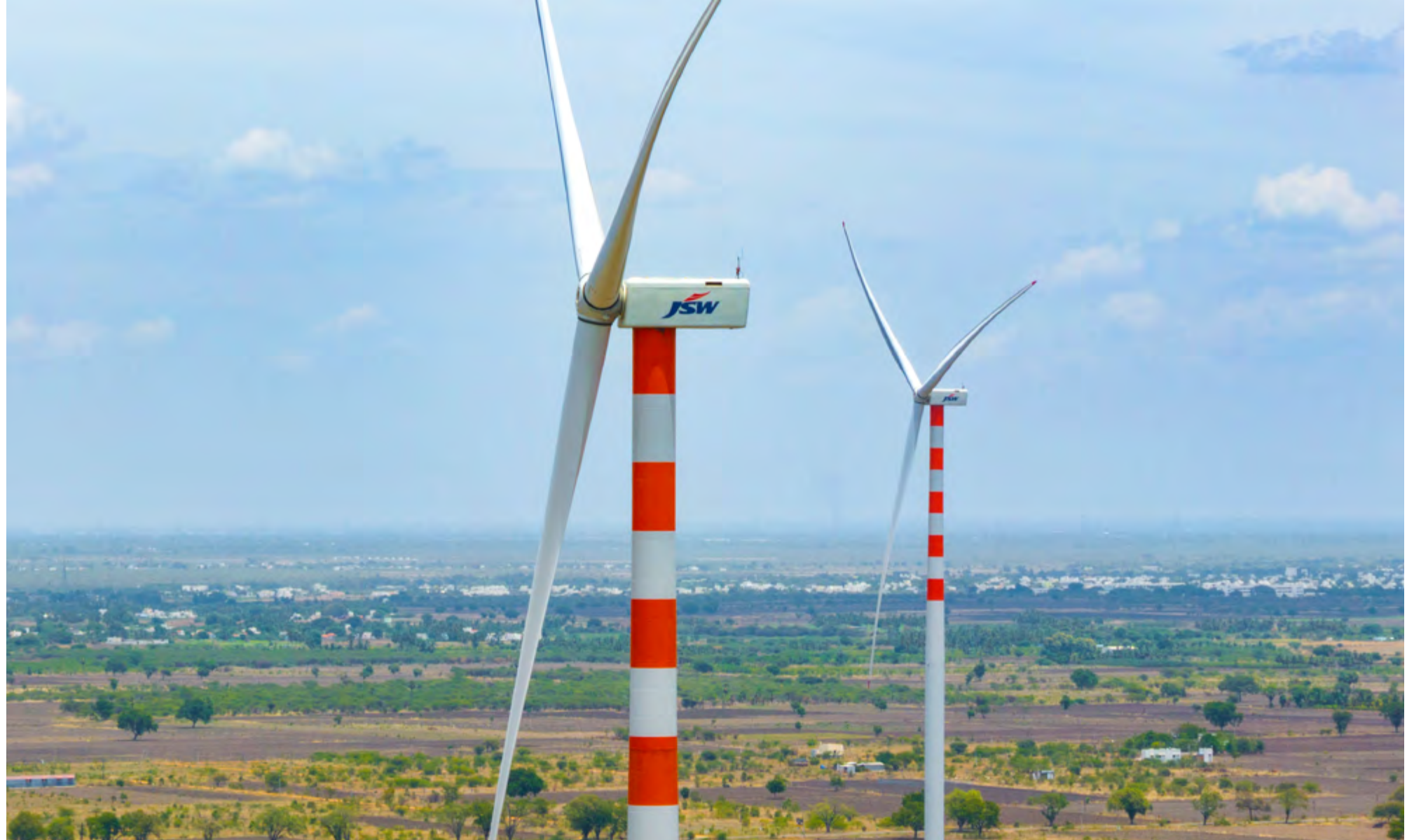
JSW Wind Energy Tuticorin Power Plant
