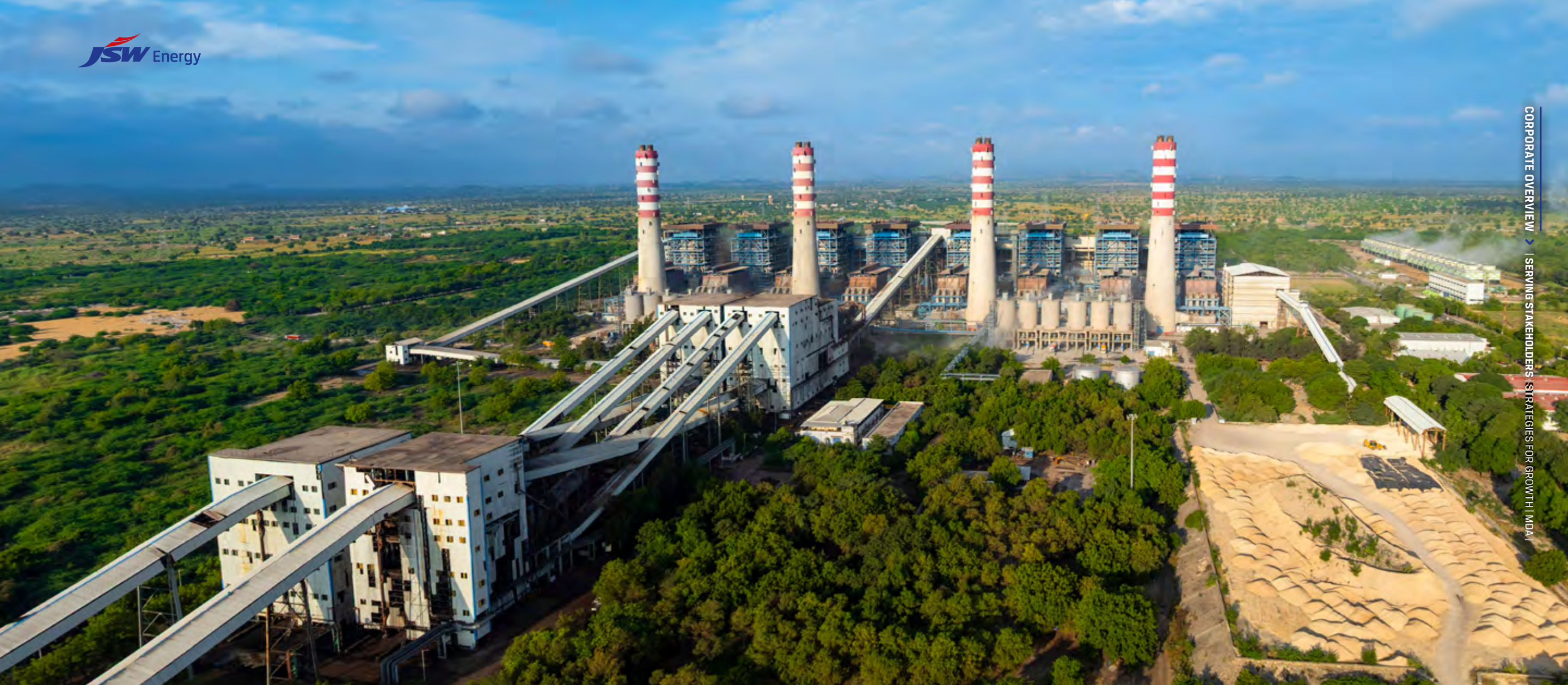
JSW Energy Barmer Power Plant
