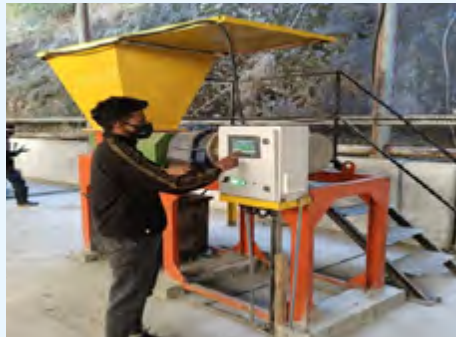
Solid Waste Management Facility JSW Hydro Sholtu
