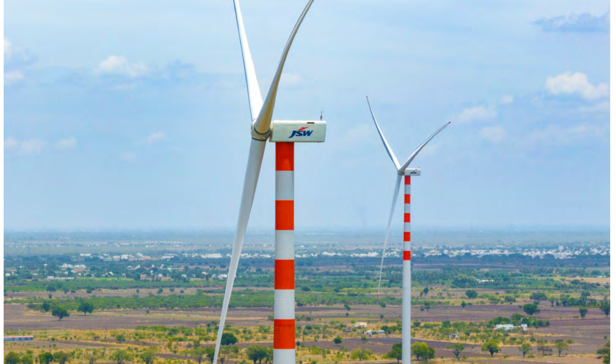
JSW Wind Energy Tuticorin Power Plant
