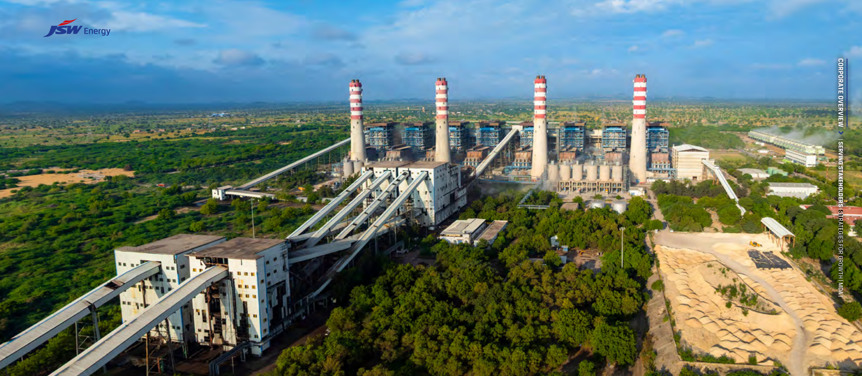
JSW Energy Barmer Power Plant
