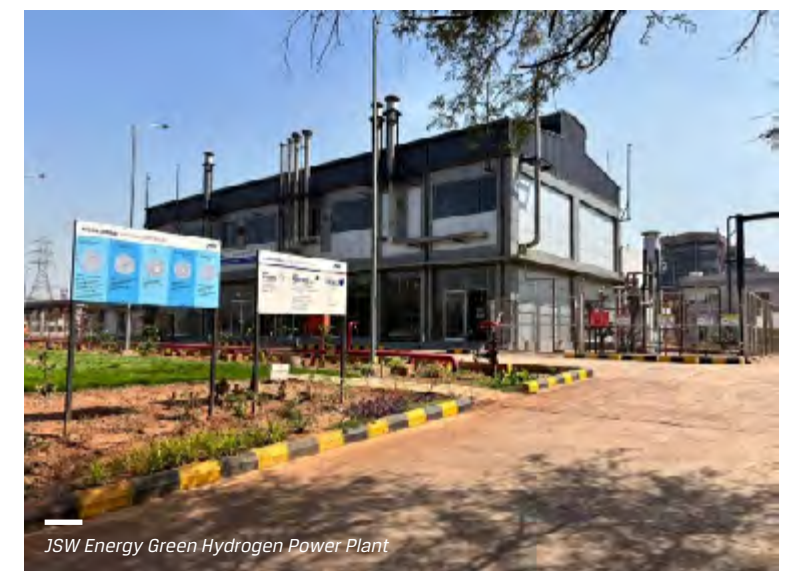
JSW Energy Green Hydrogen Power Plant
